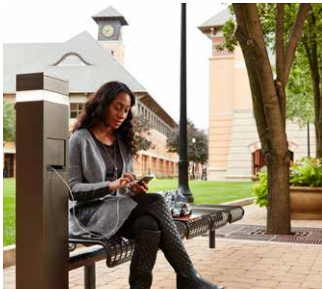
Outdoor Charging Station with Area Light.
